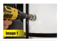
2. Remove the nut from the bulk head fitting (reversed threads) and install the agitator assembly from inside tank through the hole cut in the tank in step 1. Reinstall the nut onto the bulk head fitting and snug up to tank from the outside. Adjust the agitation assembly to a slight downward angle (Image 2). Tighten nut until the rubber seal compresses (Image 3).
